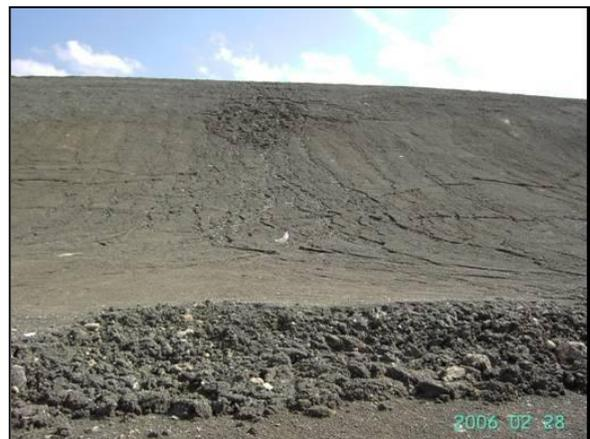
**Photo2.** Bead at the foot of the upstream slope of 14m in height
