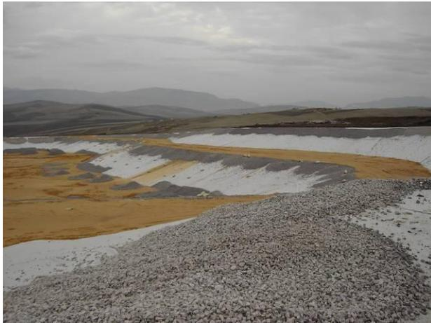
Photo 3. Receptacle with berm in construction
