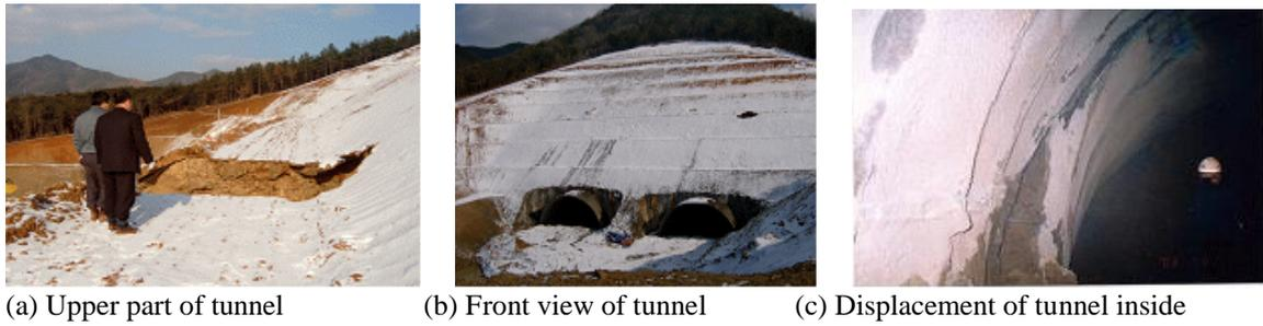
Figure 3. State of collapse zone
