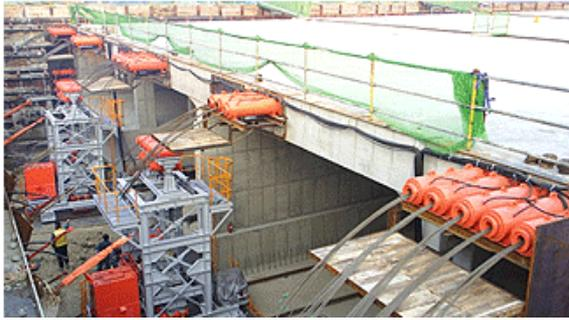
Figure 8. front jacking method
