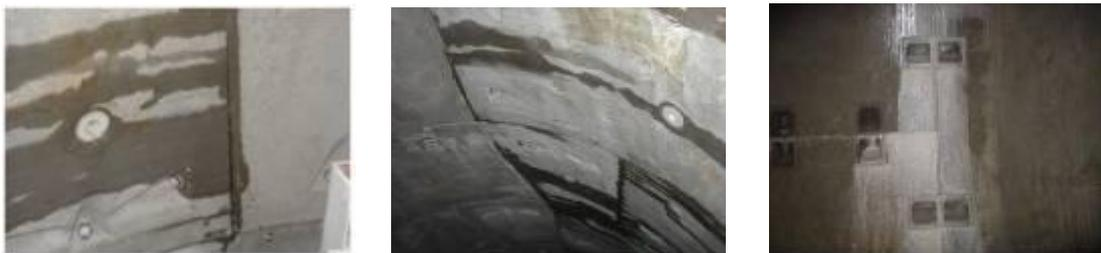
Figure 1. Occurrence of leaks of the existing segment tunnels
