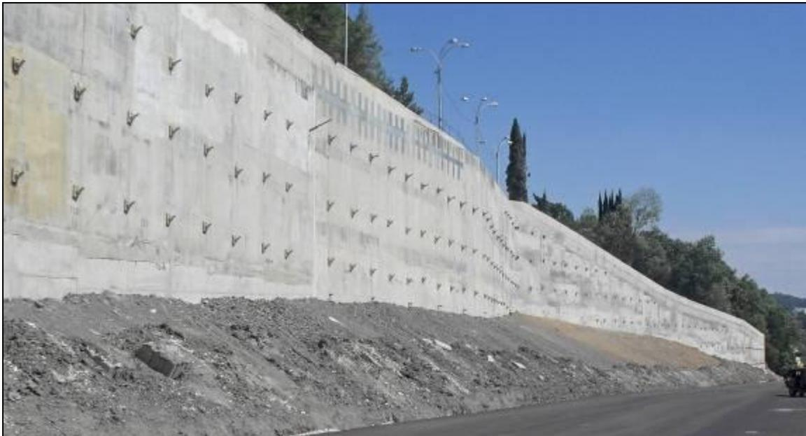
Figure 1. Pile anchor landslide protection structure at the interchange in the area of the city of Sochi
