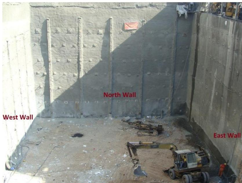
Figure 6. stabilized walls (East, North and West)
