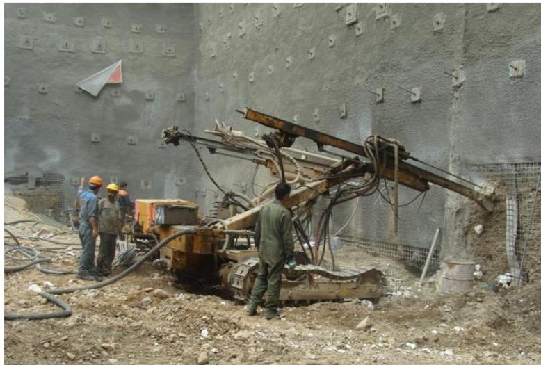
Figure 5. Drilling the excavated wall using Drill Wagon
