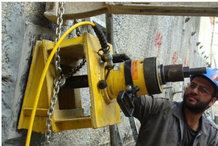
Figure 4: Posttensioning of anchors using hydraulic jack
