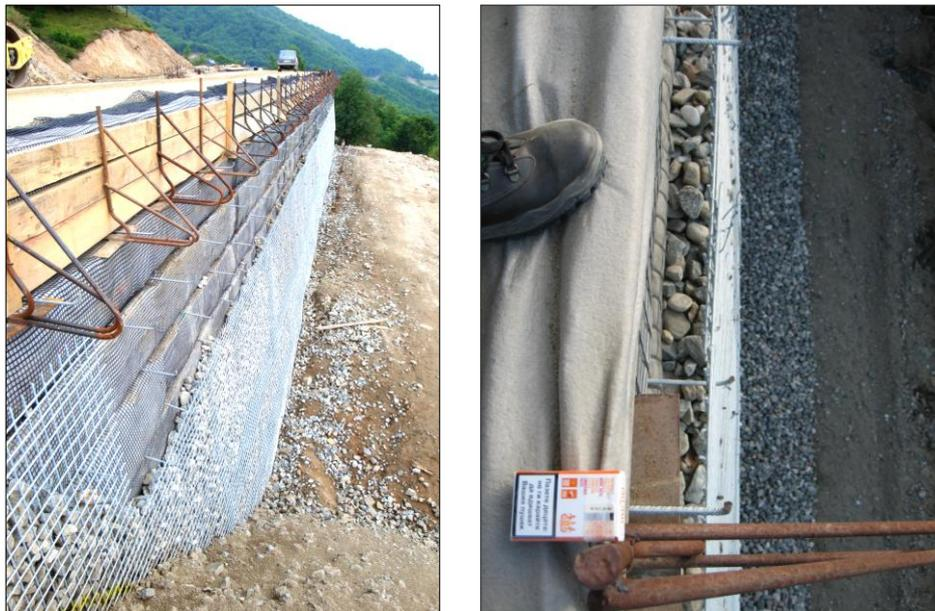
Figure 8. Left: construction stages (formwork, geogrids, anchor bars, facing), right: top view of the stone-filled facing used
