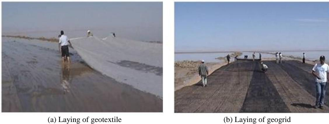
Figure 2. Installation of geosynthetic in the sabkha.
