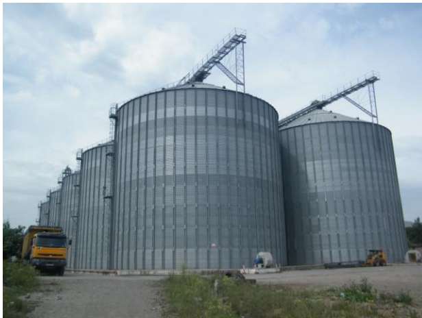
Figure 8. View of the silos.
