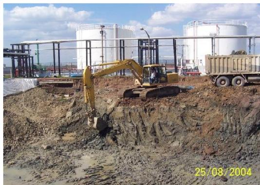
Figure 5. Excavation of existing weak subsoil (The adjacent cylindrical tanks are located in the background).
