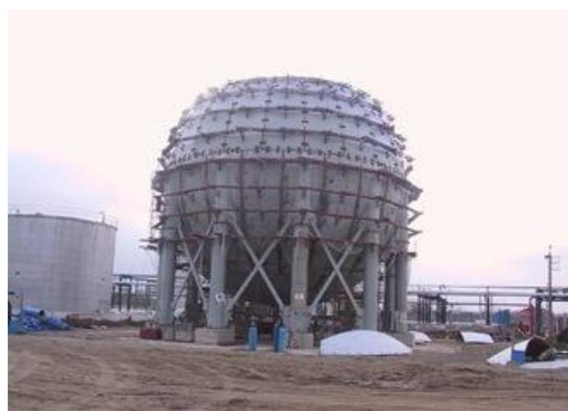
Figure 8. The sphere tank short before the final assembly.
