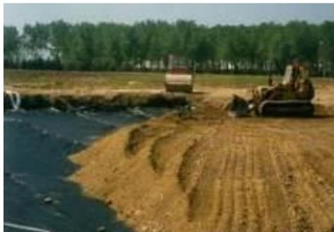
Figure 4. Production of the reinforced granular fill layer.
