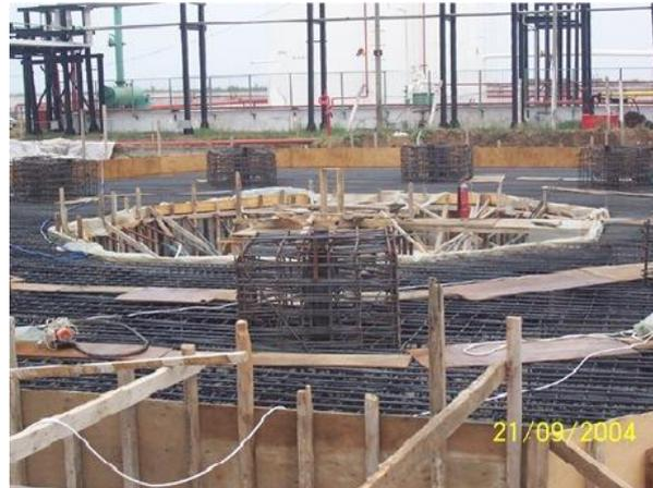
Figure 7. Installation of the reinforcement of ring foundation.
