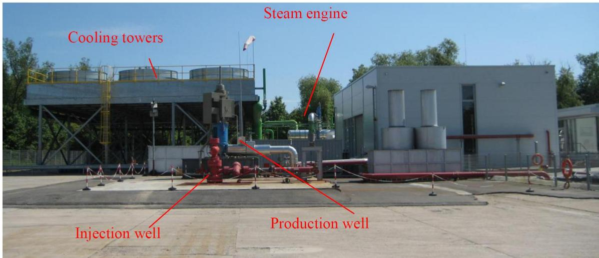
Figure 1. Geothermal power plant Landau
